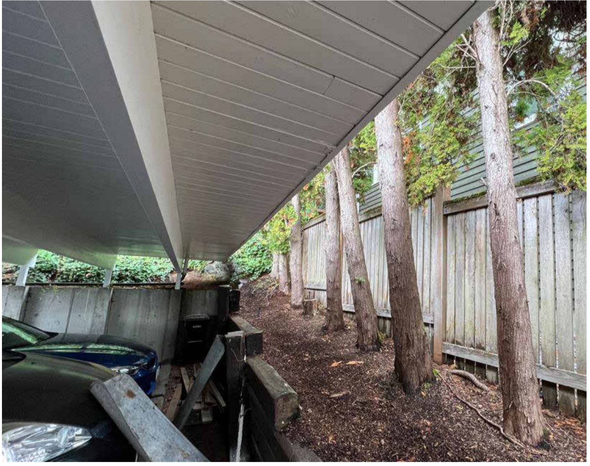
VIEW OF EXISTING NORTH RR TIE RETAINING WALL
