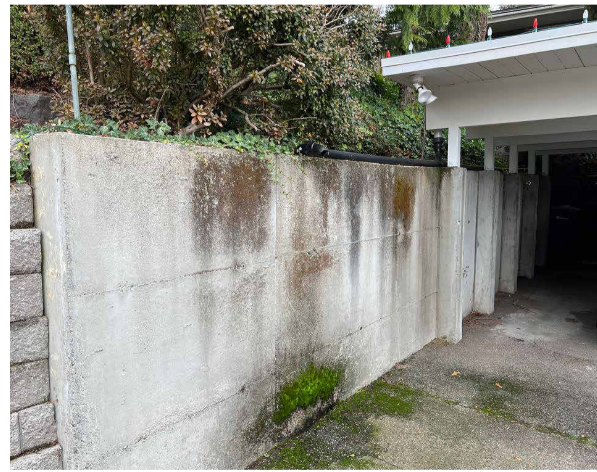
VIEW OF EXISTING WEST RETAINING WALL
